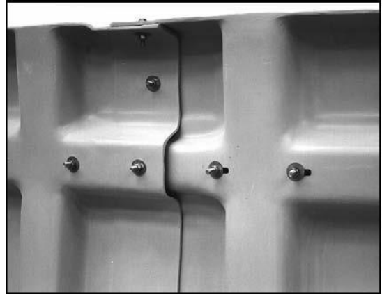
FIGURE 4: Top Flange Bolt Detail
