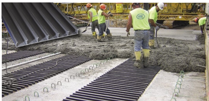
SAFPLANK®, when turned upside down, serves as an excellent concrete forming system in applications where corrosion and weight are construction concerns.
