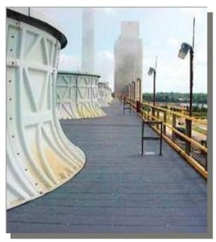
Star Cooling Towers decking system panels interlock and overlap to form a safe, strong working surface on your cooling tower. Manufactured of pultruded fiberglass reinforced polyester, the lightweight, high strength and corrosion-resistant design offers quick, easy installation. It is available with a gritted surface for fan decks and hot water basin applications.
