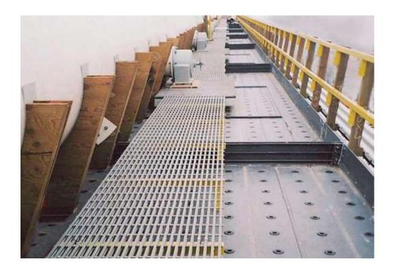
Star Plank hot water basin panel system interlocks and overlaps to form a safe, strong working surface on your cooling tower.
