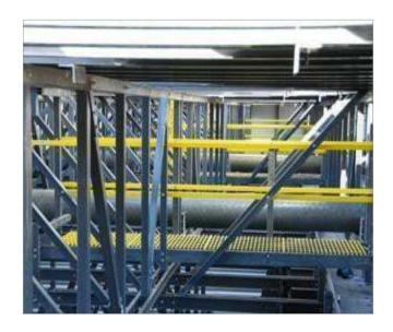
Star Cooling Towers offers fiberglass equipment access walkways and work platforms for permanent or temporary use. They are corrosion-resistant, slip-resistant, ultraviolet-resistant, strong, lightweight, and fire-retardant.
