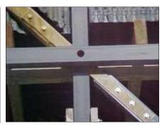
Star Cooling Towers pultruded fiberglass structural shapes allow you to replace deteriorated wood columns, beams, and decks on your cooling towers with strong, lightweight, rot-resistant fiberglass.
