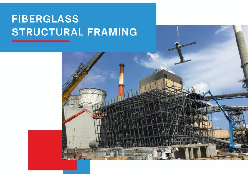
Design wind loading is in accordance with ASCE 7 for the wind velocity and exposure for the new cooling tower location. Pultruded polyester resin structural fiberglass shapes for columns, braces, joists, and ties are in accordance with CTI Standard-137 "Fiberglass Pultruded Structural Products" and CTI Guideline ESG-152 Structural Design of FRP Components".
